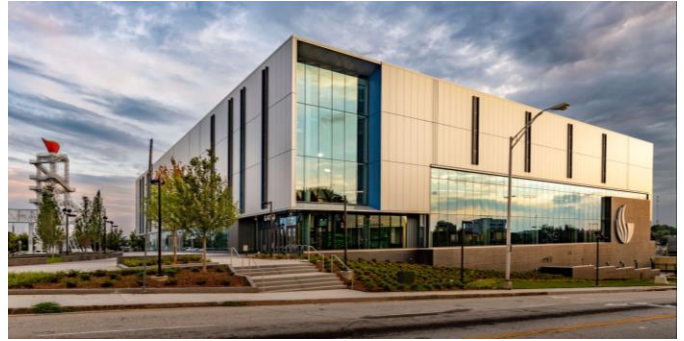
Georgia State University – Atlanta, GA Designed by Perkins & Will. The Convocation Center is a community catalyst — turning an inward-focused campus outward on civil rights grounds. The Summerhill Master Plan revitalized a long-neglected intown neighborhood. $3.2B annual economic impact.
