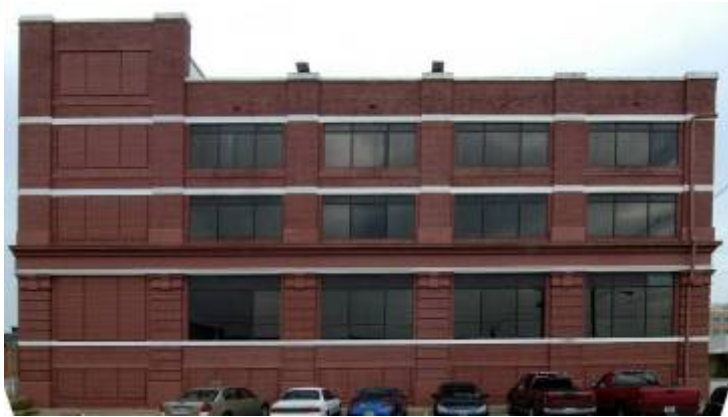
McKee Street Building Facade
