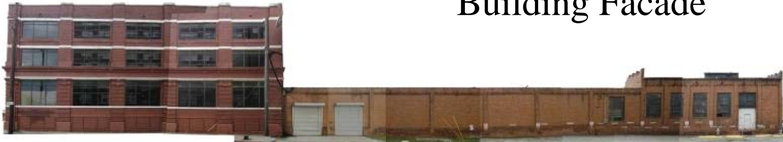
Arnold Street Building Facade
